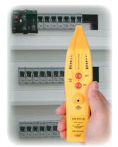
The Circuit breaker that supplies the Transmitter circuitry is the one, that (when pointed out by the tip) has the most LEDs lit on the bar-graph and the fastest buzz.
